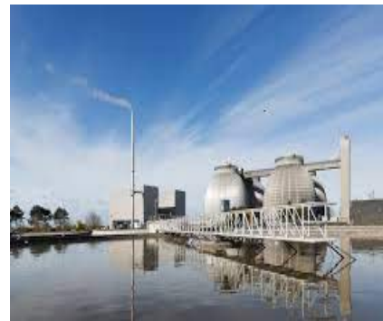
BIOFOS, City of Copenhagen Denmark
